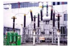
Functions and use: The technology and equipment can be used for the regeneration and purification of transformer oil, insulating oil, lubricating oil, hydraulic oil, turbine oil, fireresistant oil and engine
