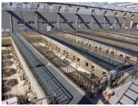
Functions and uses: MBR is used for wastewater treatment. Technical indicators: new technologies such as gas impulse and mechanical cleaning are integrated into the membrane unit; a variety of techniques controlling the filterability of the mixed liquor enable the extension of the membrane operation cycle by 2-4 folds; online chemical cleaning modes are suitable
