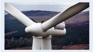
carbon fiber used as a reinforcing material in large wind turbine blades, the performance parameters of the blades see remarkable improvements, which are mainly manifested as follows: As the stiffness increases, the weight decreases; 2. The power output of the wind turbine is more smooth and stable; 3. The manufacturing, transportation and installation costs of the wind turbines are reduced
